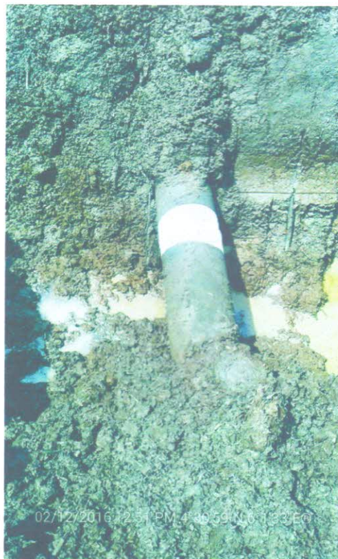
Incident Point after Repairs
